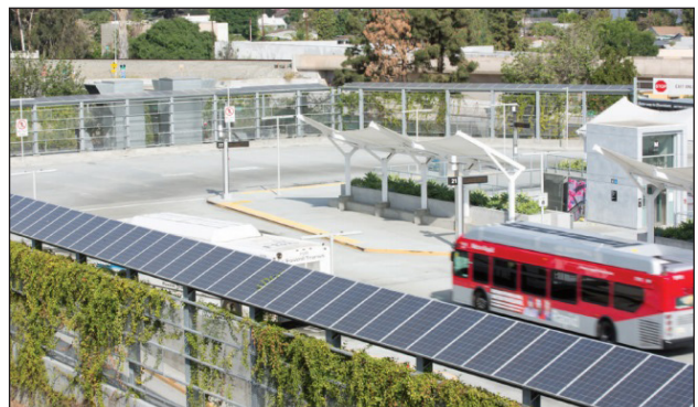
Figure 2-1 Solar Panels at El Monte Station.
