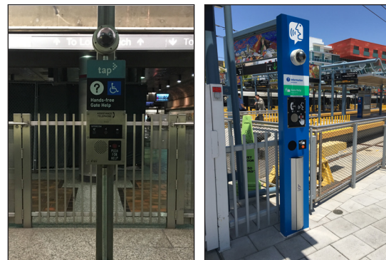
Figure 1-2 Gate telephones on the B (Red) and E (Expo) Lines.
