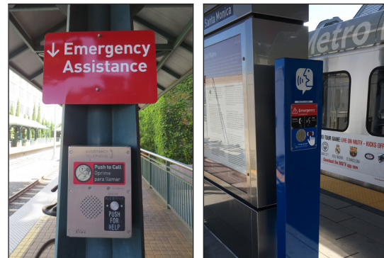
Figure 1-1 Emergency telephones on the L (Gold) and E (Expo) Lines.
