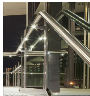
Figure 3-6 Integrated handrail LED pods basis of design with inset detail.
