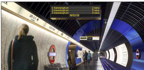
Figure 3-4 Platform edge linear LED downlight example, TFL.
