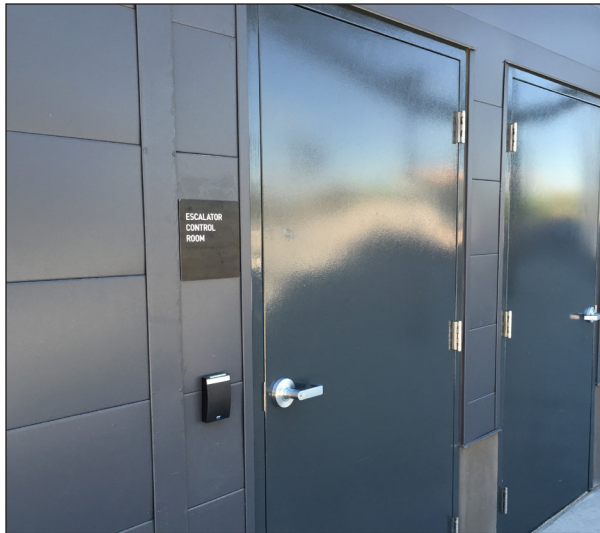
Figure 3-3 Escalator controller located in a nearby room, behind and under the escalator at Universal/Studio City Station, B (Red) Line.
