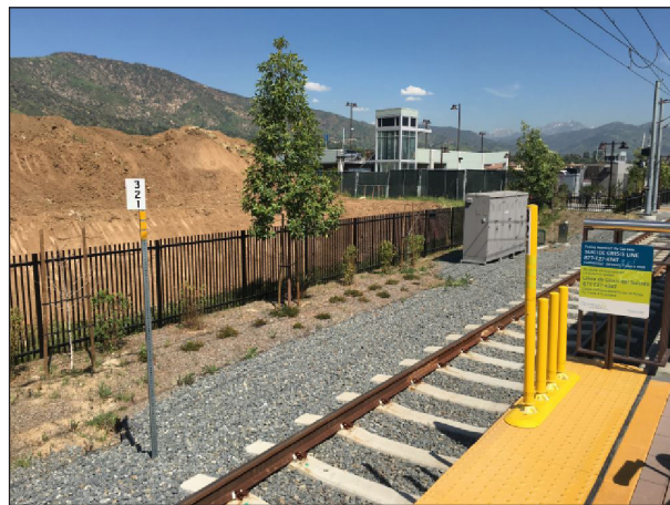
Figure 1-2 Existing ad-hoc berthing marker installation on tracks at APU/Citrus College Station, L (Gold) Line.
