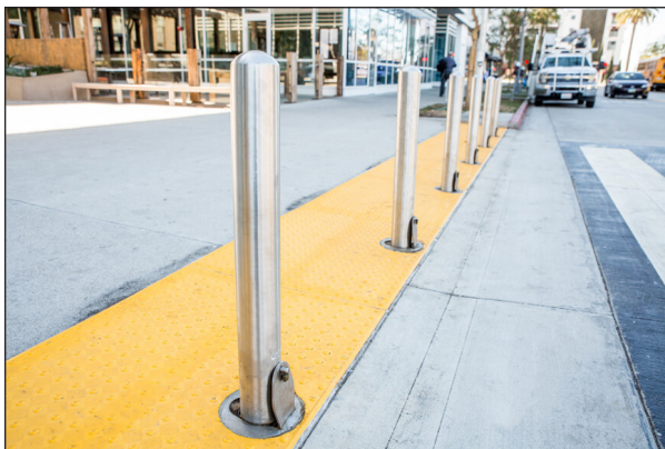
Figure 2-1 Stainless steel operable bollards with dome tops.
