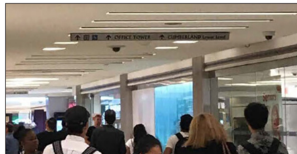
Figure 2-3 Security camera flush to ceiling with matching finishes.
