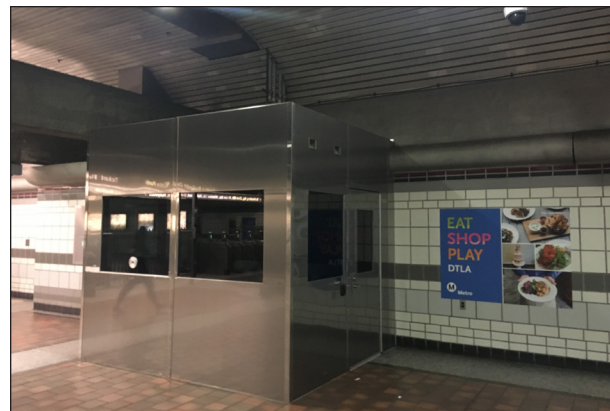
Figure 1-2 Kiosk with tinted windows located in corner, away from passenger activity, 7th St/Metro Center station, B/D (Red/Purple) Line.
