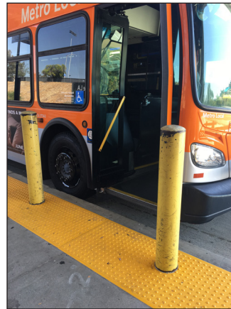
Figure 1-1 Painted VSBs that need to be repainted and maintained, Cal State LA station, J (Silver) Line.
