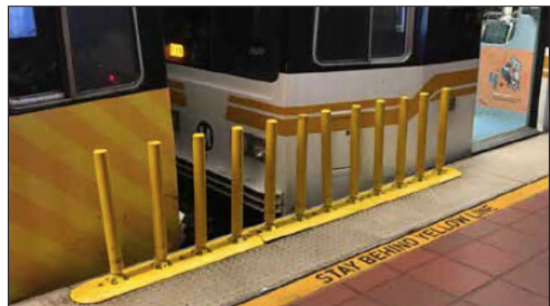
Figure 1-5 Between-car-barriers located on platform edge. A (Blue) Line platform at 7th St/Metro Center station.
