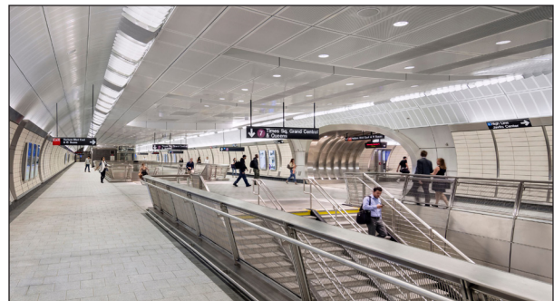
Figure 2-1 Integrated materiality. 34 St-Hudson Yards station, NYMTA.
