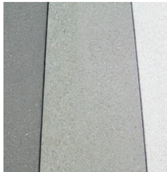
Three-tone Concrete Paving
