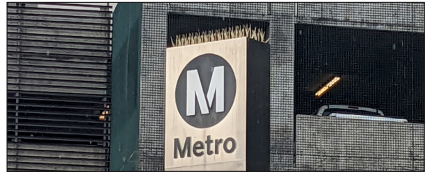
Figure 1-2 Bird spikes on a pylon sign, Pershing Square Station.
