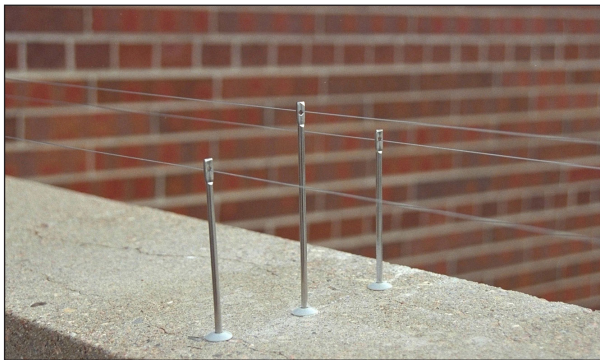
Figure 3-6 Example bird wire system installation.
