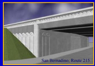
Developing Aesthetic Treatment Options and Themes Structural Design Elements: Slope Paving Examples
