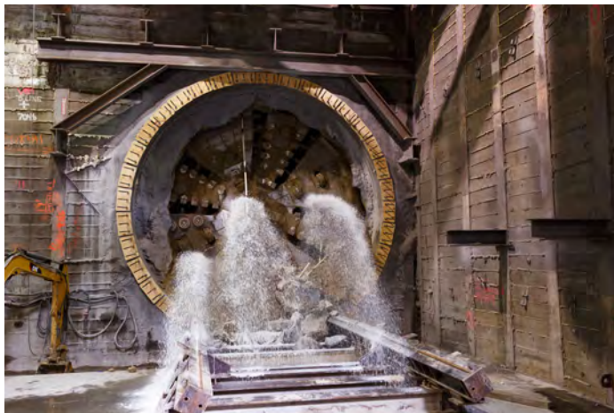
Tunnel Boring Machine at Leimert Park Station
